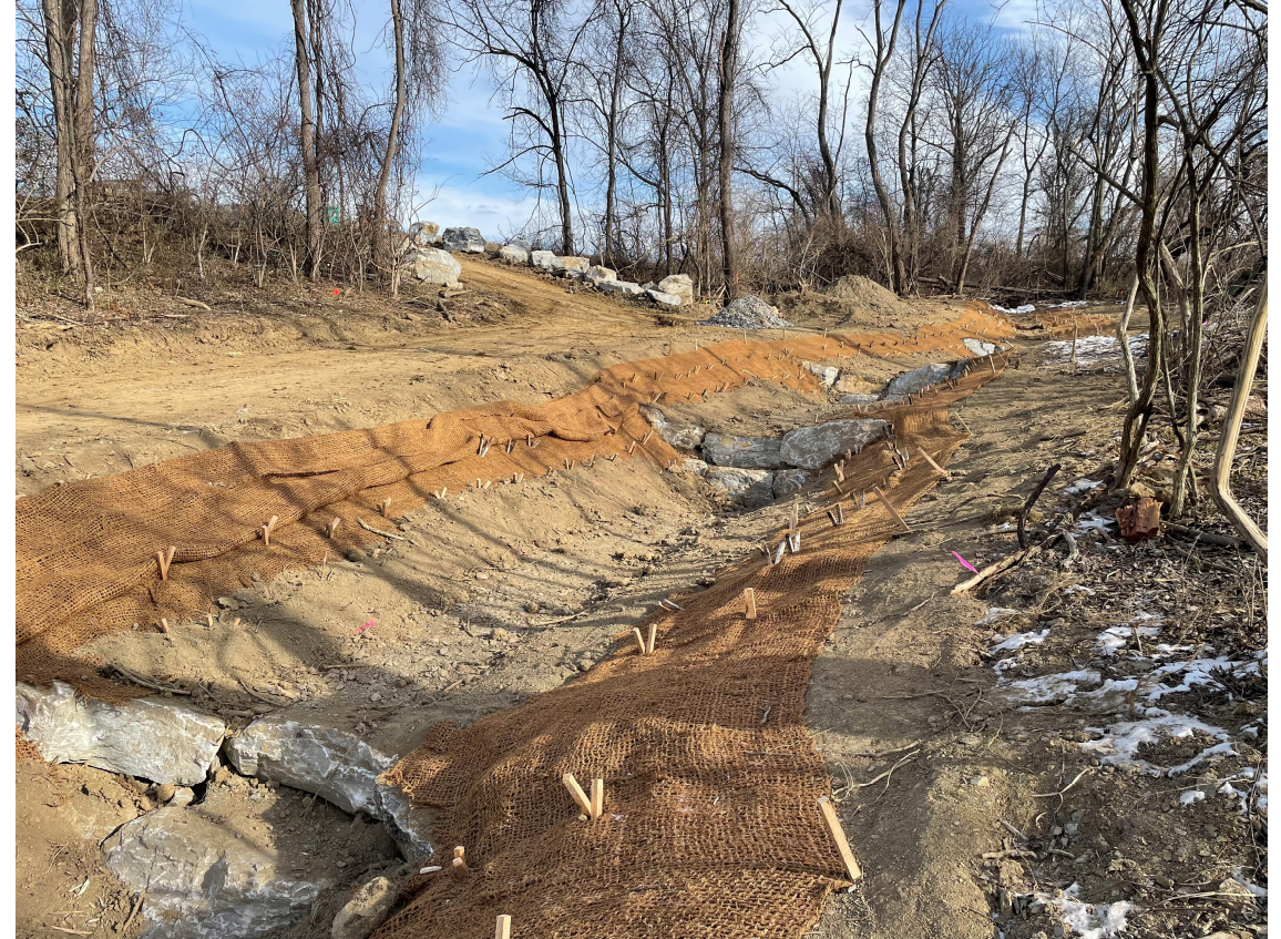
Facing northeast/upstream of Reach 1 and Reach 2 Rock Steps with Erosion Control Matting
