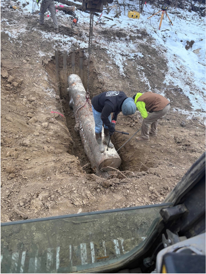
Installing Reach 1 Log Step
