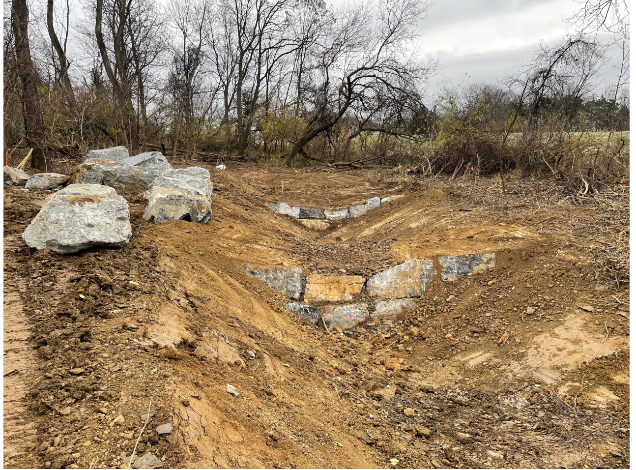
Installing Reach 1 Rock Steps
