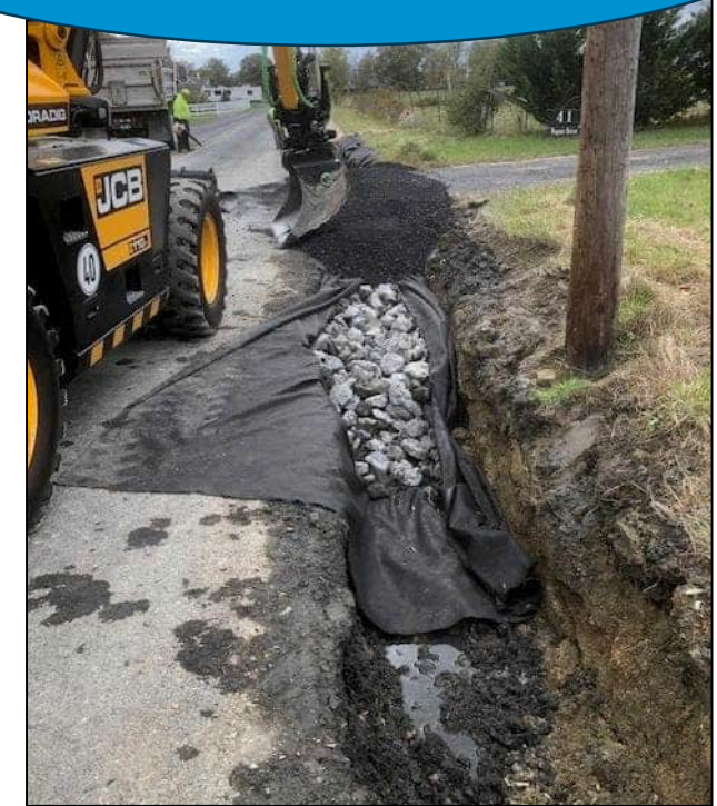
Project 2 during construction at the east end along Wagner Drive
