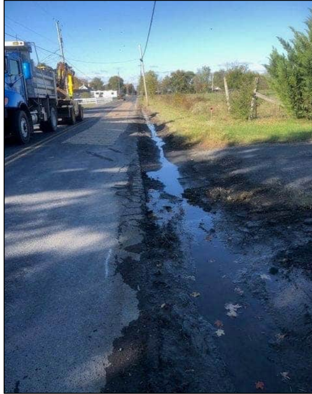
Project 2 before construction at the east end along Wagner Drive
