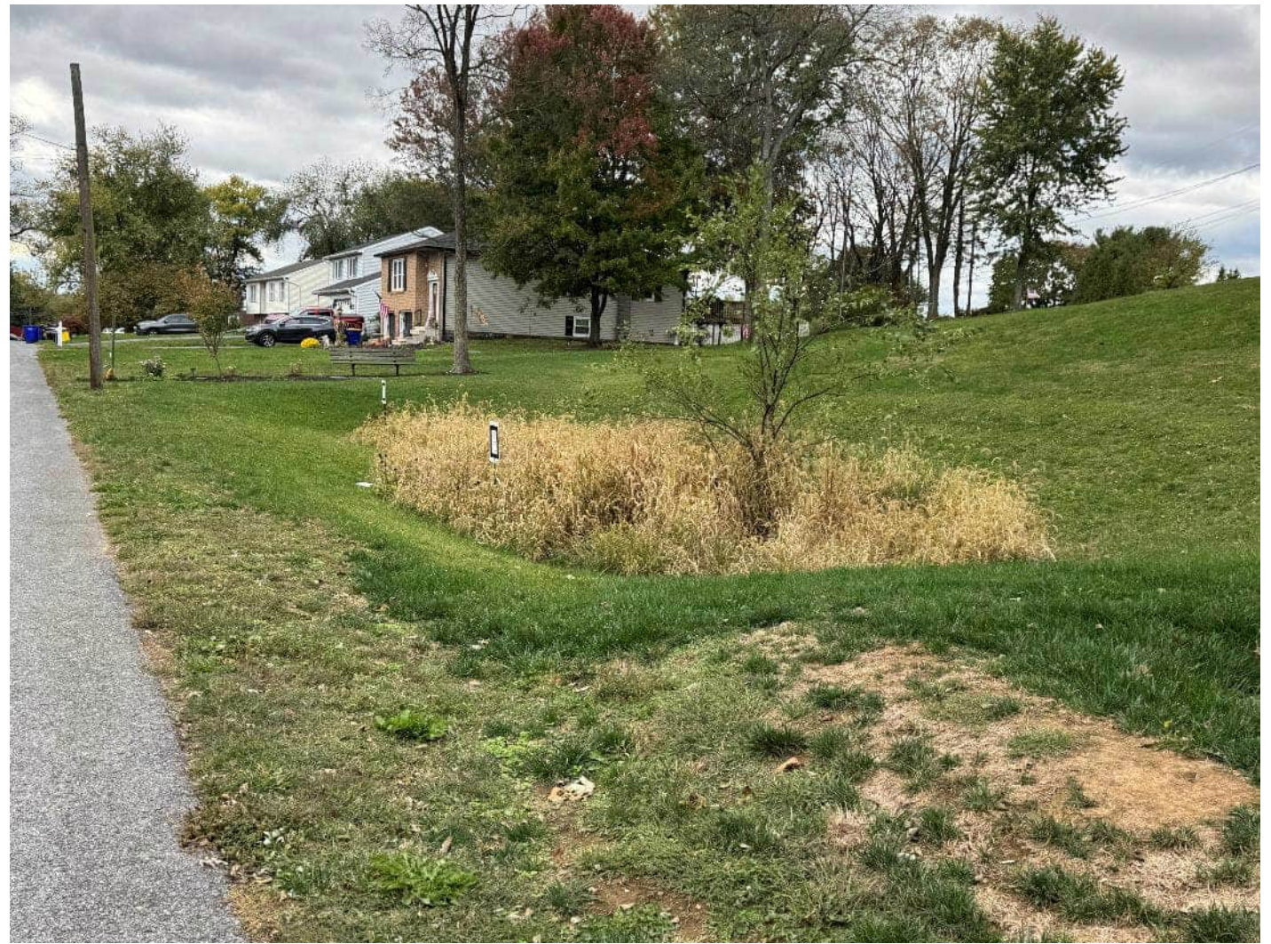
Project 7 rain garden at Anderson Park post-construction one year later
