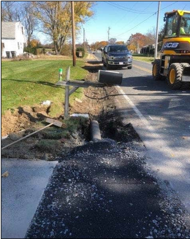
Project 1 Wagner Drive near the western end during construction
